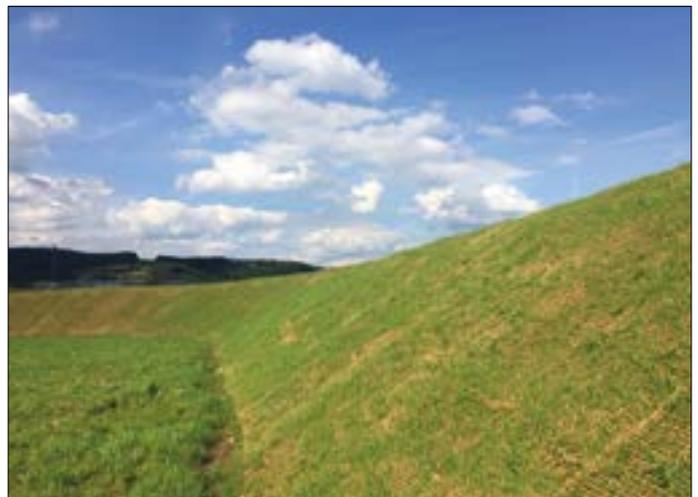
Figure 9: Coir nets on a slope
