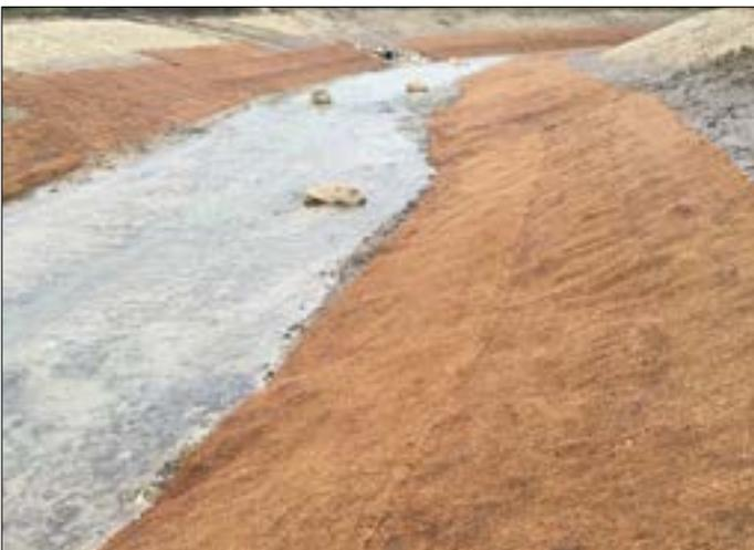
Figure 8: Coir nets in trenches and brooks
