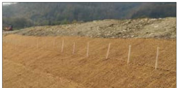
Figure 5: Installing the coir net with wooden fixings
