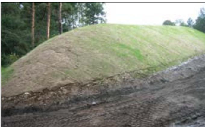
Figure 8: Jute nets on a slope
