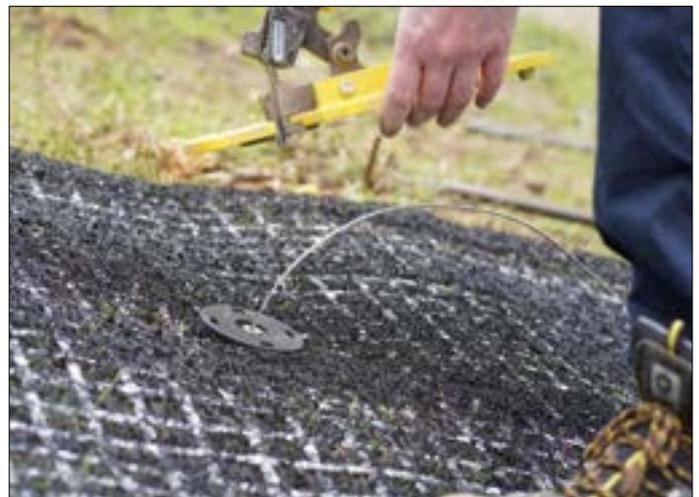
**Figure 5:** Loadlocking and tensioning the earth anchor
